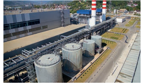
Electrical power plant
